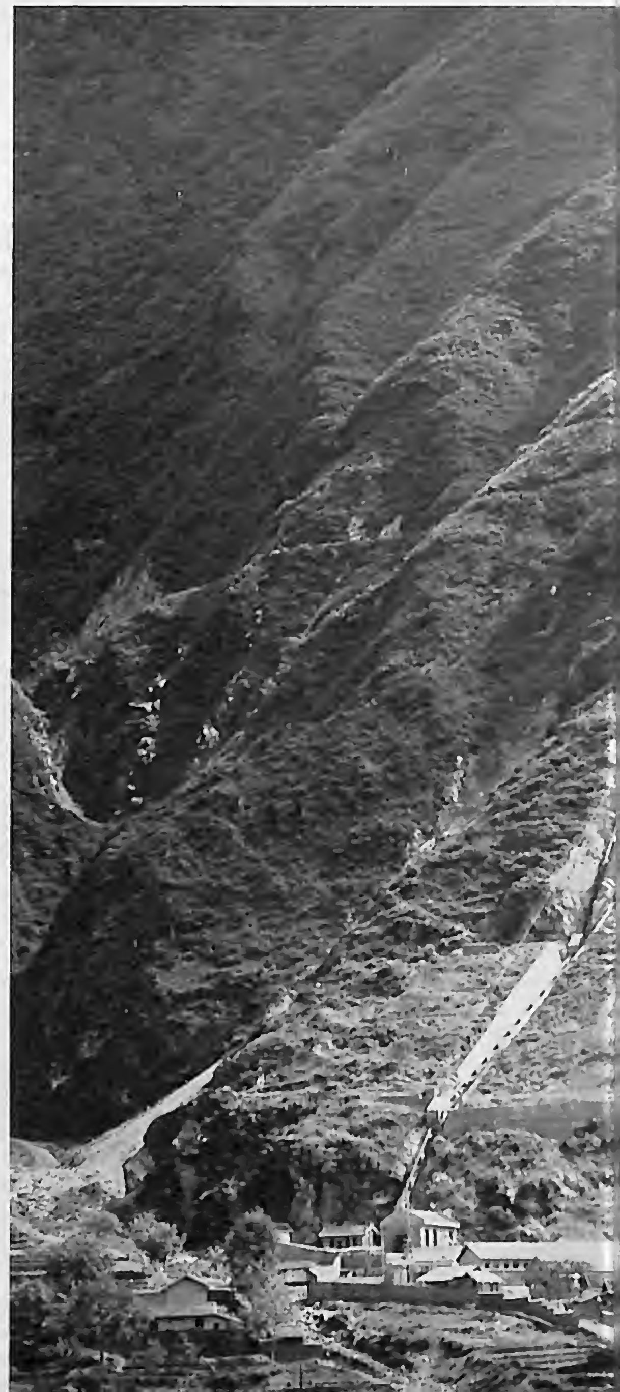
The newly-built Luting Hydro-Power Station.
